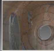
Dirt on the inside of the outer tub
